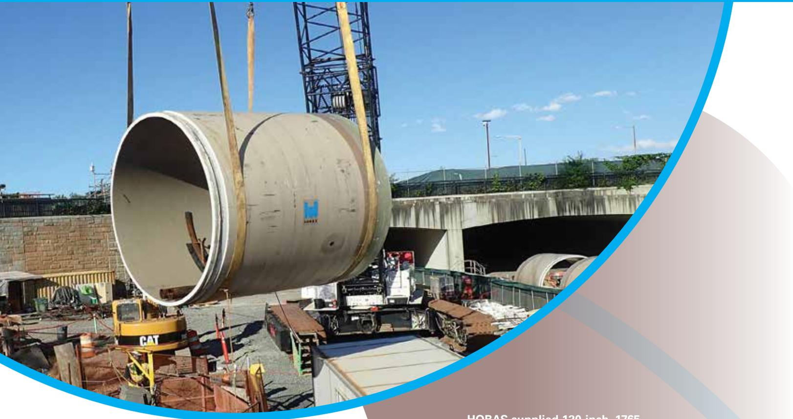
**HOBAS supplied 120-inch, 1765-ton jacking pipe for this project although 600 tons of jacking force was all that was needed to complete the drives.**
