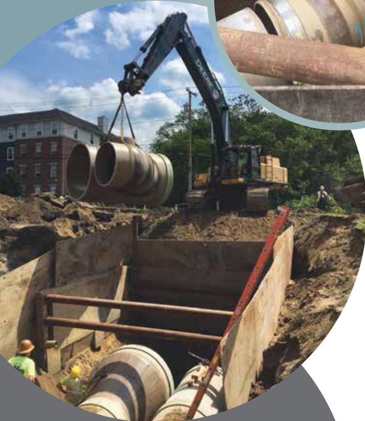
A large wye is lowered for connection to the already installed CCFRPM pipe. The lightweight pipe requires less equipment and is easy to maneuver on the job sites.
