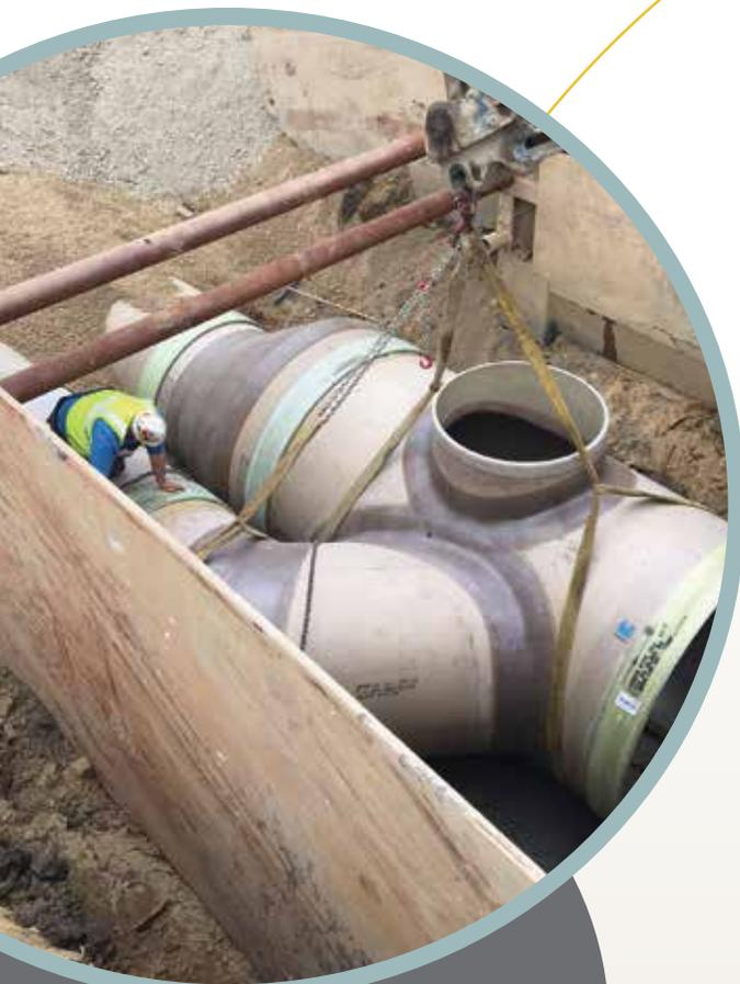
These fittings are manufactured of the same materials as CCFRPM pipe and almost any mitered fitting can be constructed. Here a wye with a tee base has been custom manufactured per job specifications.
