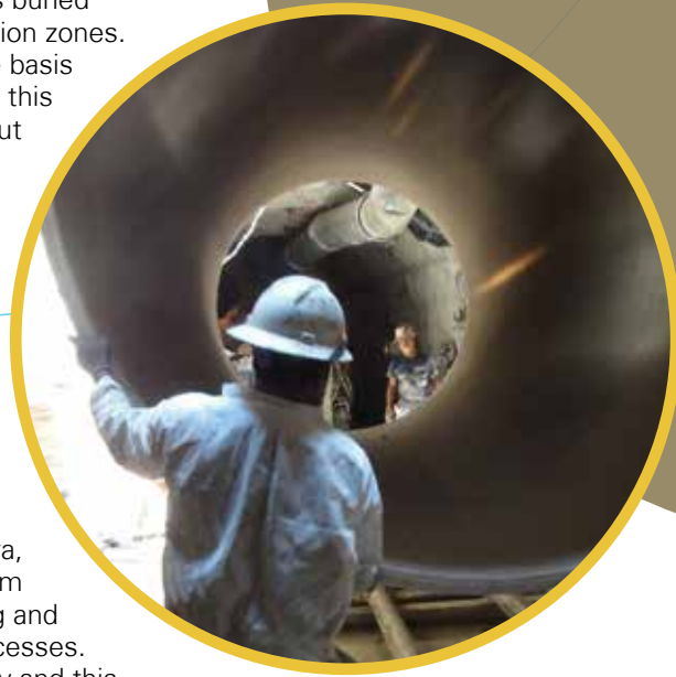
With tunnel depths reaching 50 to 80 feet, future repairs would prove difficult. Designers wanted a corrosion resistant material leading them to choose HOBAS CCFRPM.
