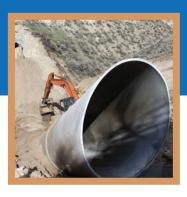
**Direct Bury:** HOBAS is the preferred pipe for deep installations and withstands covers in excess of 80 feet.
