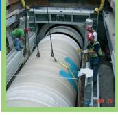
Sliplining: The smooth interior surface and oversized I.D. typically maintain or increase flow capacity. Low profile and flush bell-spigot joint options give you a choice of joint configurations.
