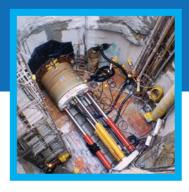
Microtunneling or Jacking: HOBAS pipe's high strength and smooth, constant O.D. permit drives of 500 to 1,000 feet with lower force and fewer jacking stations.
