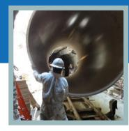
Tunneling: Two-pass tunneling requires a smaller primary tunnel because of HOBAS high strength, thin-wall pipe. This reduces excavation and spoil removal. Longer insertion pushes speed installation and require fewer shafts. HOBAS pipe can navigate curves, too.
