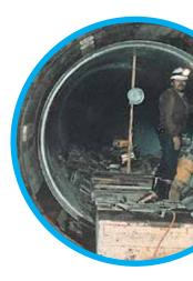
**Tunneling:** Two-pass tunneling requires a smaller primary tunnel because of HOBAS high strength, thin-wall pipe. This reduces excavation and spoil removal. Longer insertion pushes speed installation and require fewer shafts. HOBAS pipe can navigate curves, too.
