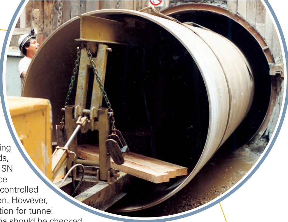
Lightweight HOBAS pipes transport easily into the tunnel.
