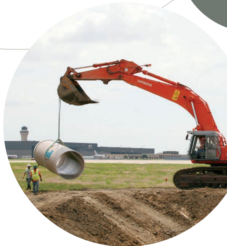
Direct bury installation at DFW Airport
