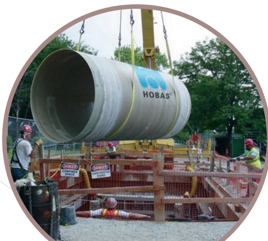
FIGURE 17 - Pipe Insertion
