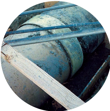
Joining HOBAS pipes (left) to ductile iron with a HOBAS FWC coupling.
