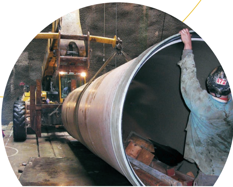
60-inch diameter, 100 psi sewer force main in a two-pass system.
