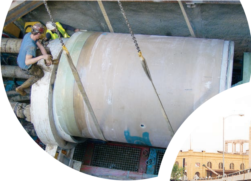
84-inch diameter jacking pipe for the City of Los Angeles.
