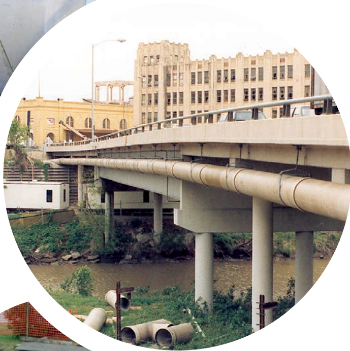
30-inch diameter sanitary sewer vent line.
