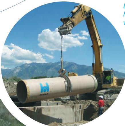
*Lightweight HOBAS pipes handle easier and lay faster with less expensive equipment.*
