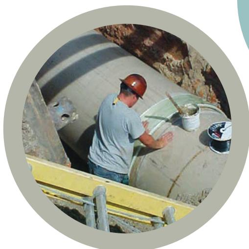
*HOBAS push-on FWC coupling joints assemble easily and provide leak-free service.*
