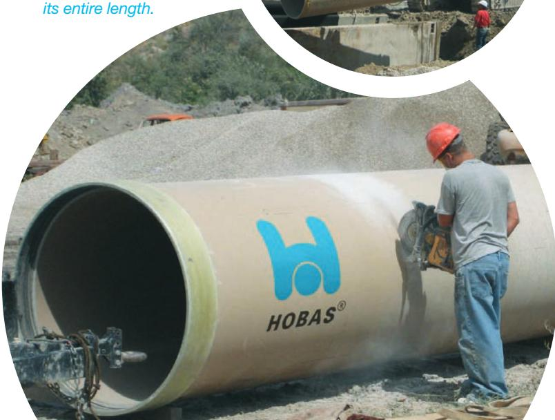
*Smooth, constant OD of HOBAS pipes permits cutting and joining anywhere along its entire length.*
