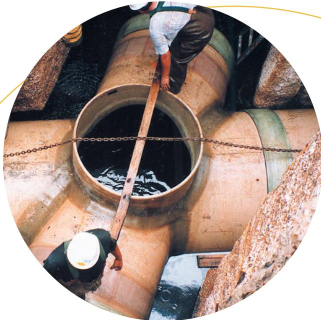
*Almost any fitting configuration and angle can be constructed with HOBAS fiberglass reinforced polymer mortar pipe.*
