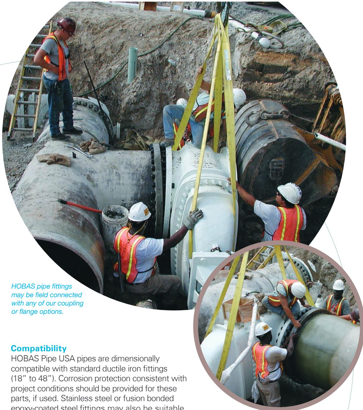
*HOBAS pipe fittings may be field connected with any of our coupling or flange options.*
