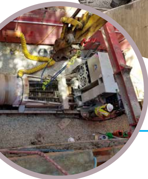
The pipeline is constructed by consecutively pushing pipe and the MTBM through the ground using a jacking system for thrust.
