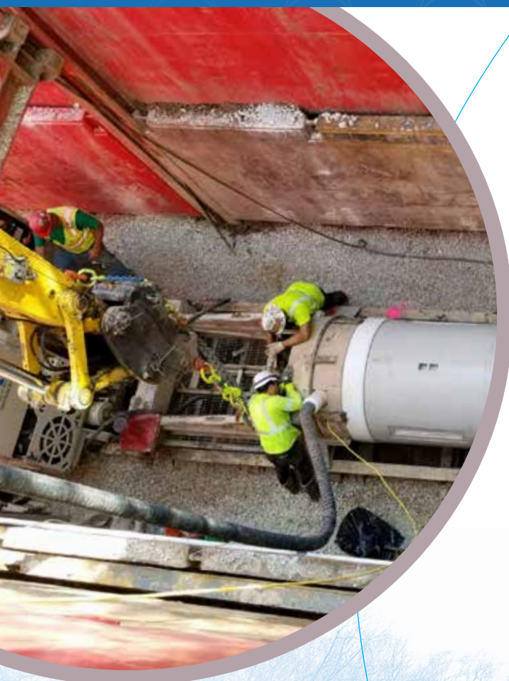
A microtunnel boring machine (MTBM) will help to maintain a precise line and grade for the new pipeline.
