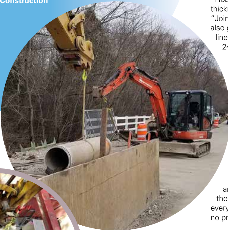
The pipeline is constructed by consecutively pushing pipe and the MTBM through the ground using a jacking system for thrust.
