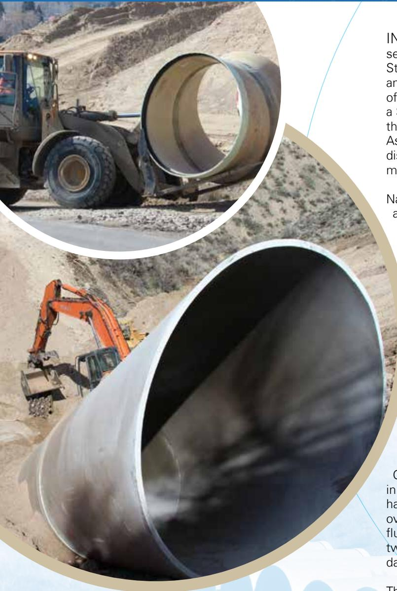
*The existing wood stave flumes were replaced with 96-inch inverted siphons made of Hobas Pipe.*
