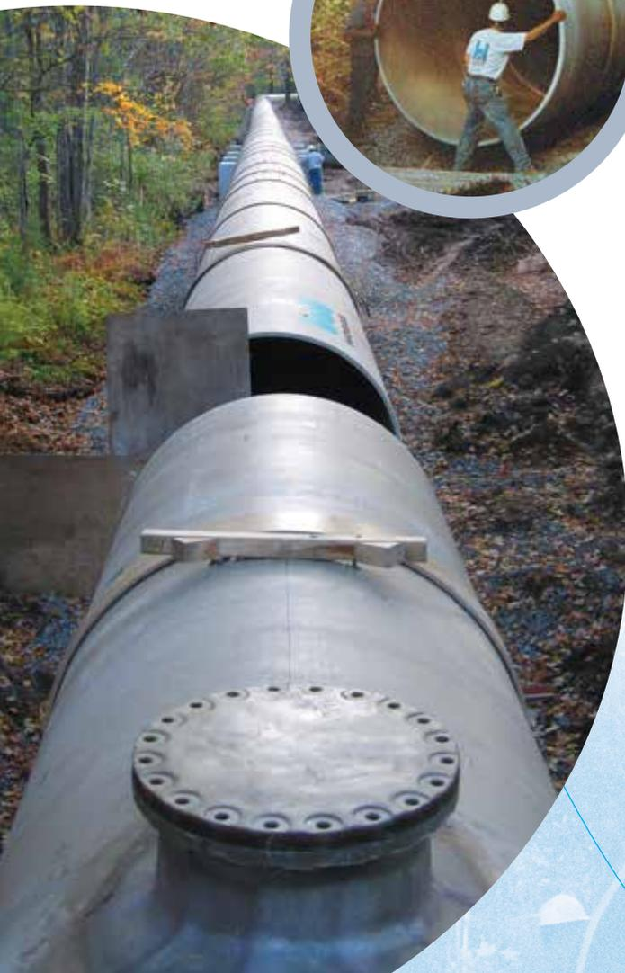
MEANDERING THROUGH THE WHITE MOUNTAINS, a large wooden penstock served as the main water supply for a local hydro facility. Jackman Station, as the facility is referred to, is fed by the Franklin Pierce Reservoir, which was created by the hydro's dam and surrounding earthen dikes. The water elevation in the reservoir is managed according to spring run-off.
