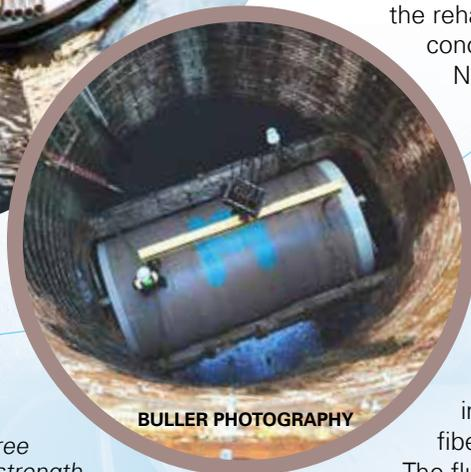
The existing tunnel was approximately 132-inches in diameter and the 120-inch CCFRPM pipe has an outside diameter of 126-inches. This allowed a clearance of only three inches which due to the high strength thin walled Hobas pipe, maximized the I.D. post rehab.
