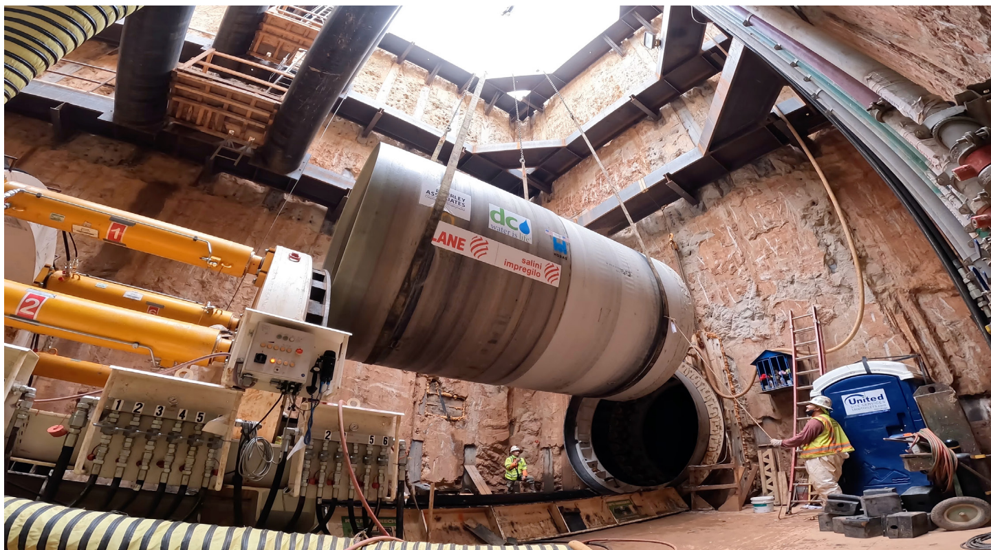
A length of Hobas pipe is moved into place in a Washington, DC, diversion sewer project. The jacking frame, at left, helped push the pipe into the new tunnel. Hobas provided 700 feet of 132-inch jacking pipe for the project.
