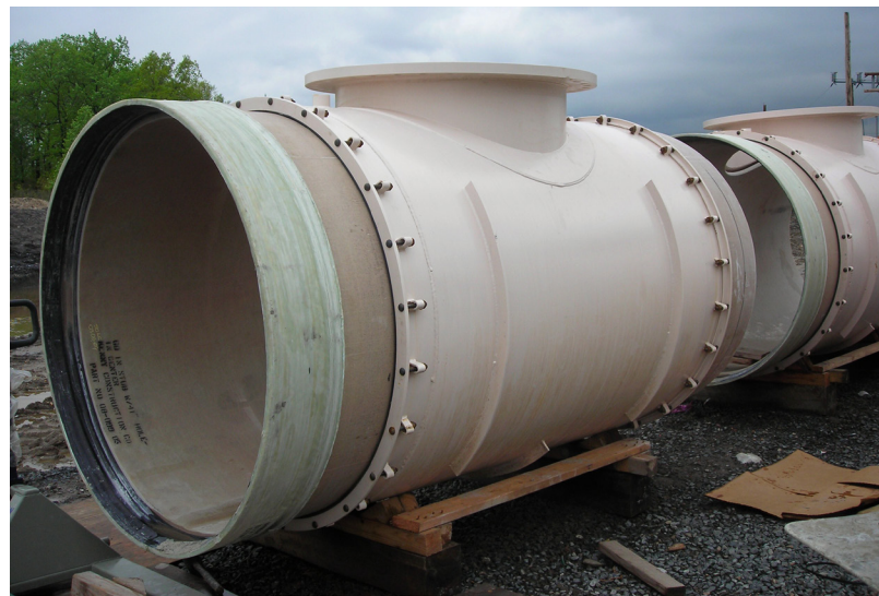
A high-pressure tee base before installation as part of an infrastructure project of the Middlesex County Utilities Authority in New Jersey.
