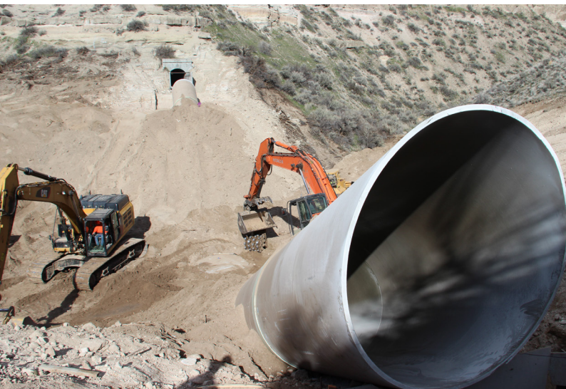
Hobas supplied a custom-built 96-inch pipe tee along with two custom elbows to create a V-shaped siphon for the Naches-Selah Irrigation District. It also supplied 3,600 feet of 96-inch pipe.
