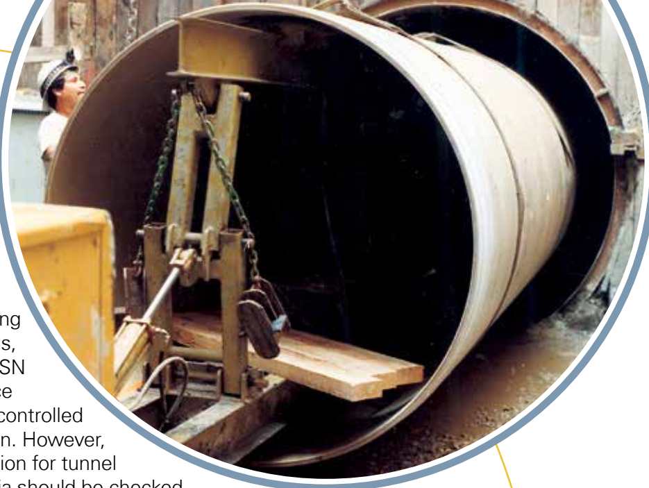
Lightweight Hobas pipes transport easily into the tunnel.
