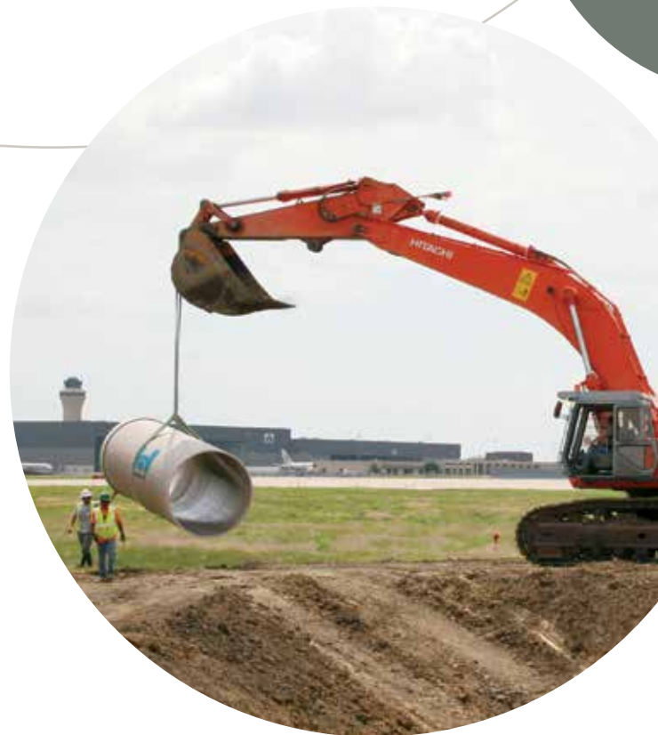
Direct bury installation at DFW Airport
