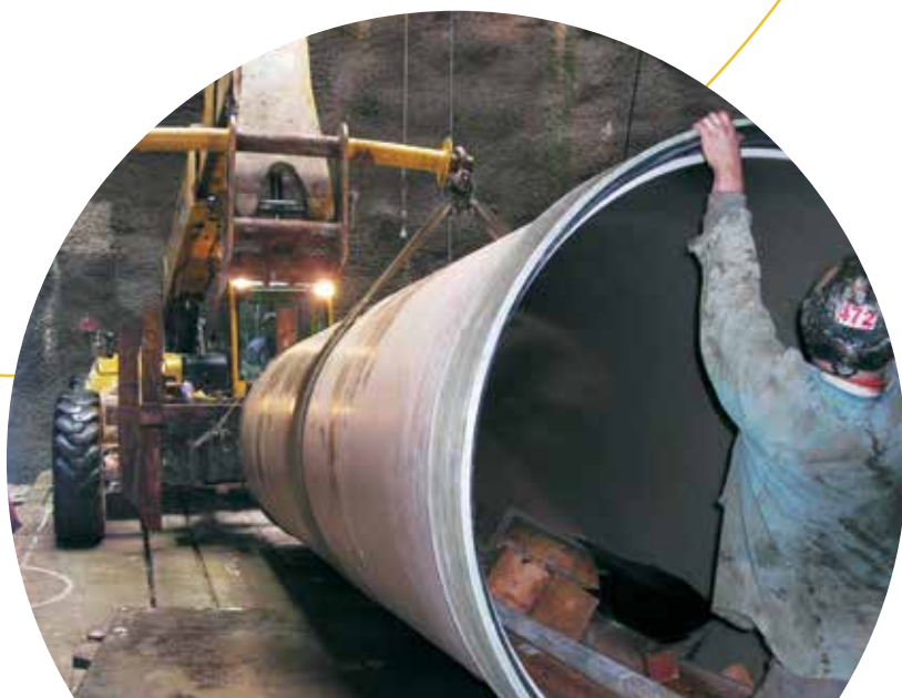
60-inch diameter, 100 psi sewer force main in a two-pass system.
