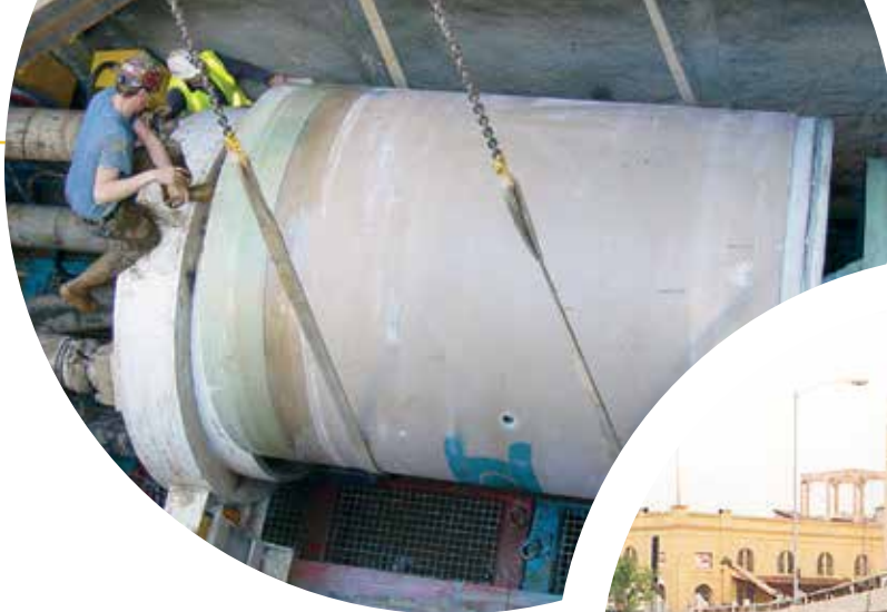
84-inch diameter jacking pipe for the City of Los Angeles.
