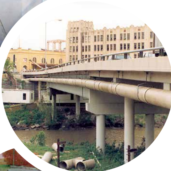
30-inch diameter sanitary sewer vent line.
