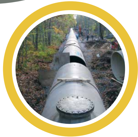
84-inch diameter Hydro-Electric Penstock in New Hampshire
