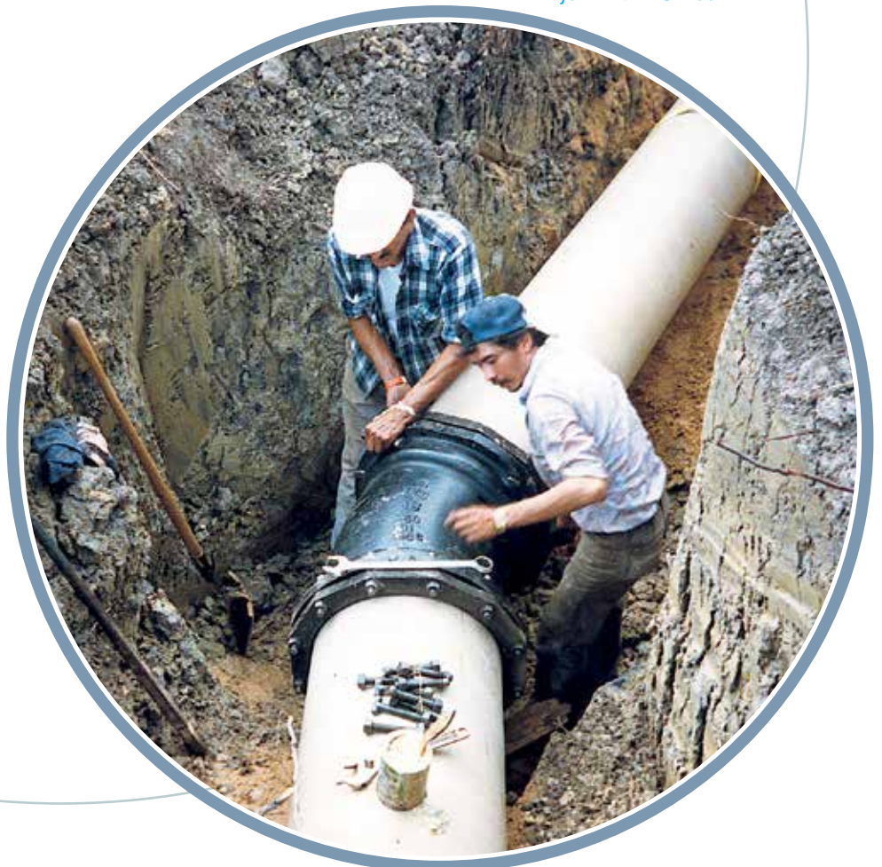
Hobas pipes' OD is compatible with DI joints from 18" to 48".
