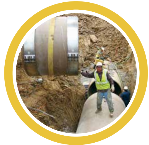
Stainless steel closure coupling.
