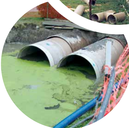
60-inch CMP storm culvert rehabilitation with 54-inch Hobas.
