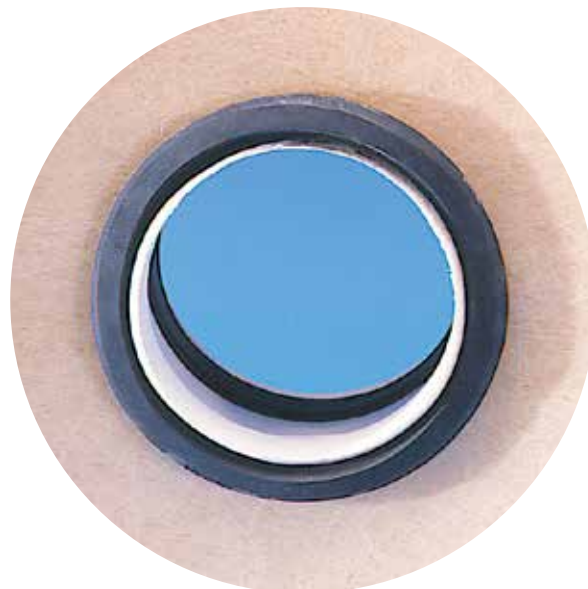
Underside (inside) of "Inserta Tee" installation.
