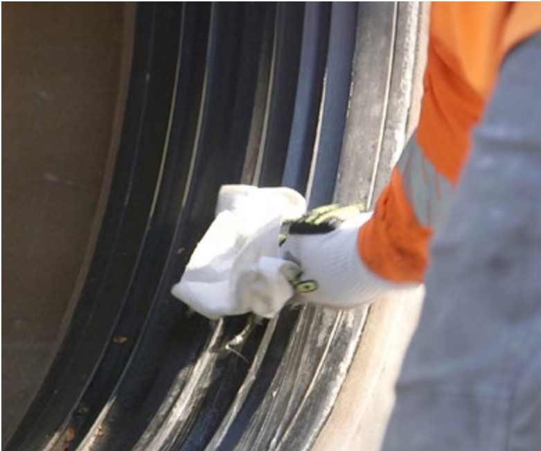
FWC coupling being prepped for installation
