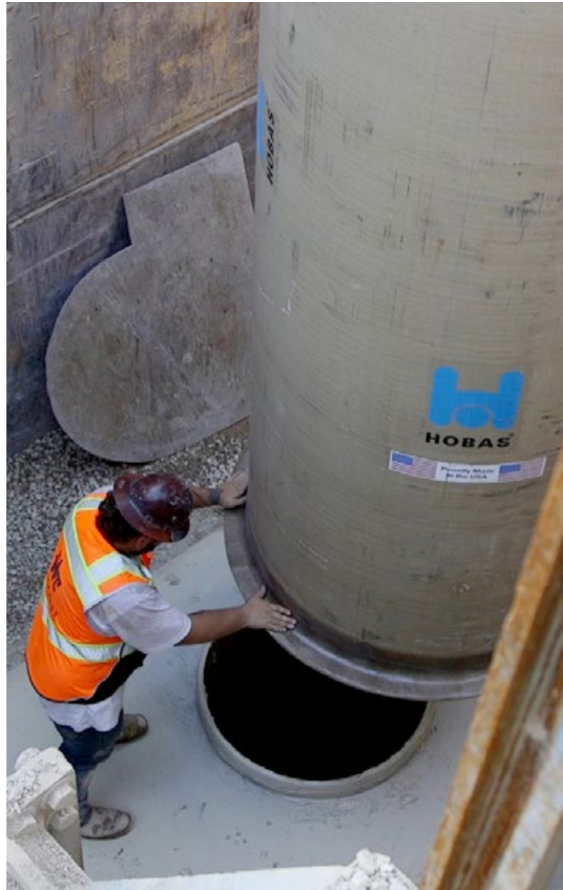
Manhole installation in Boise, Idaho.
