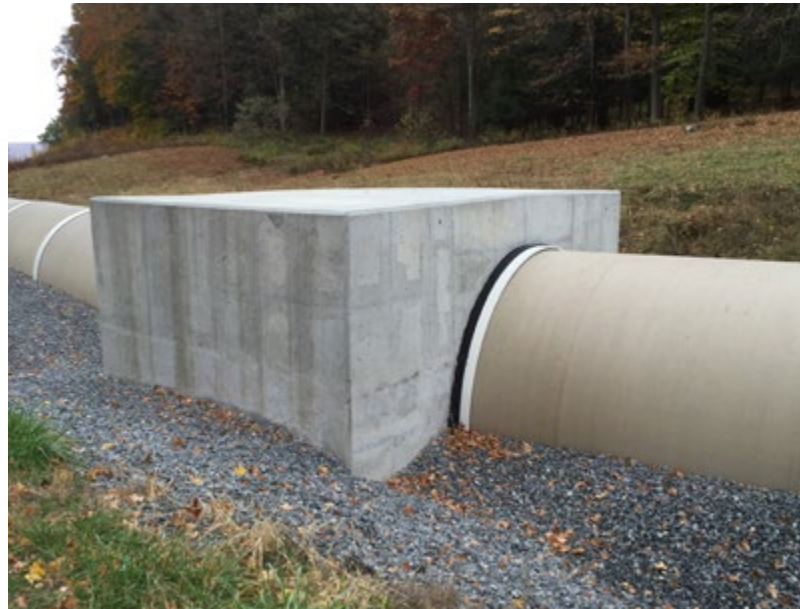
Completed NL Fitting Thrust Encasement
