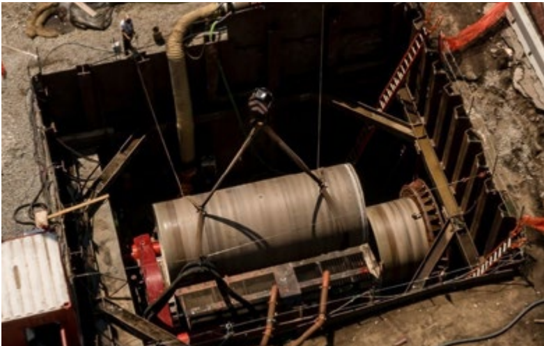
Jacking pipes have rubber ring sealed flush bell-spigot coupling for quick assembly
