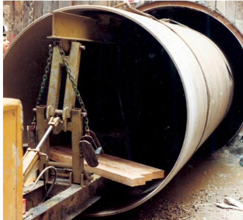
Sliplining pipe greatly extends the life of the infrastructure
