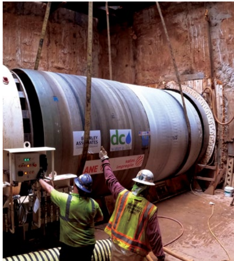
Hobas jacking pipes have the lowest drive loads
