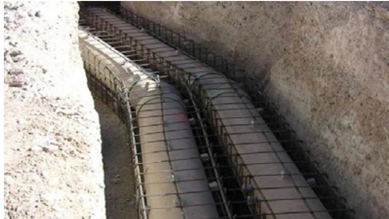
Axial concrete encasement
